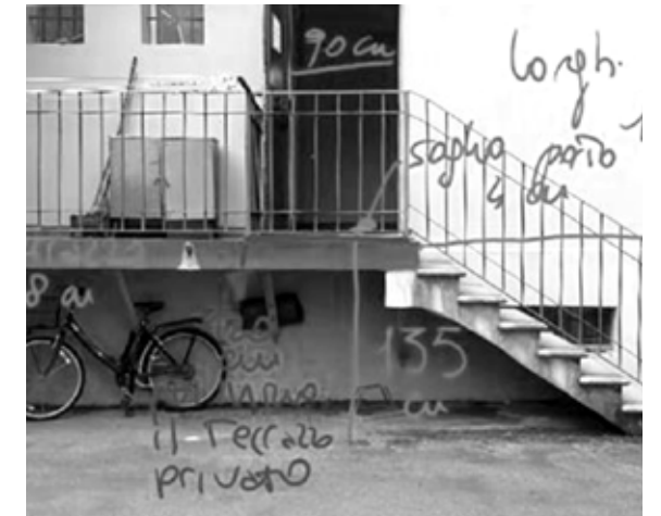
Image of some architectural notes about the accessibility of a building - CAAD
