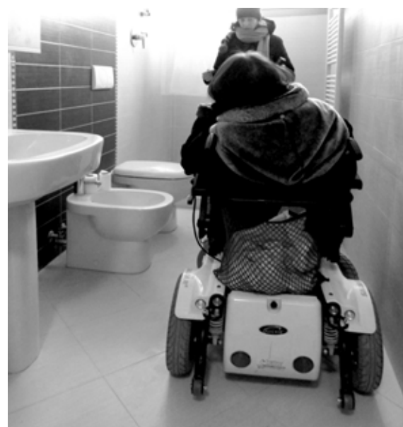
Images: home inspection and architectural analysis of a building - CAAD
