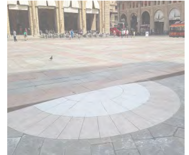
Image of “Crescentone” ramp, historical pavement of Bologna's main square
